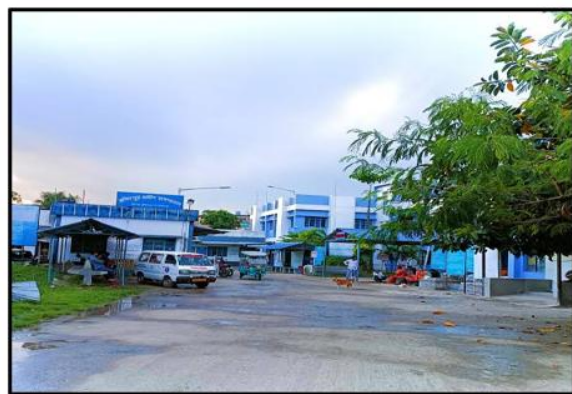
Rasidpur (Buniadpur) Rural Hospital
