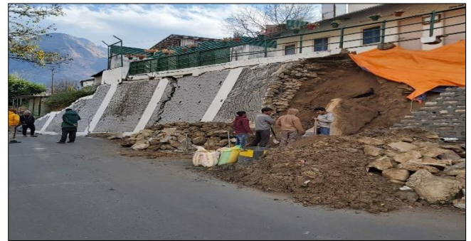
Fig 5: Fissures in boundary wall of J.P. block of hydro colony
