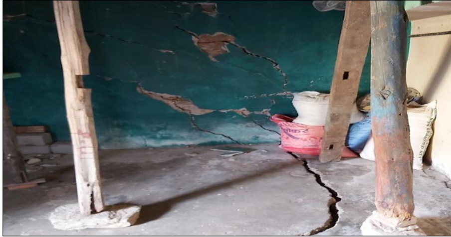
Fig 3: Cracks In A House In Joshimath
